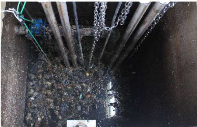
To the left, a sump tank in one of our field trials before the Flygt Concertor™ system was installed and then after two weeks of operation (right).
